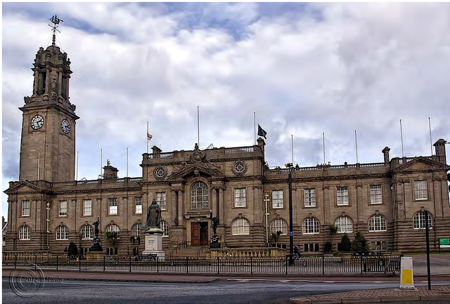
Fig.1: South Shields Town Hall
